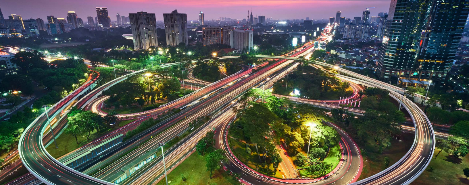
Mitsubishi Power supports the region's transition towards cleaner energy sources
